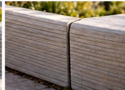
04 MODULAR ASSEMBLY Proposed segments with controlled joints
