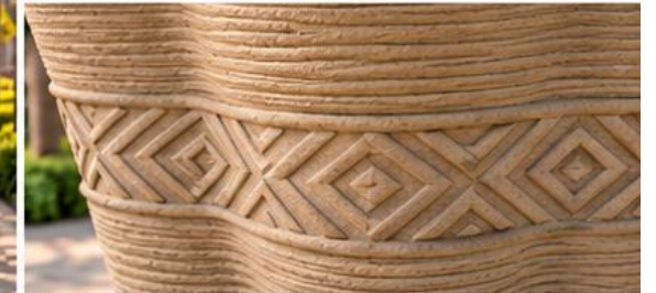
3D PRINTED CONCRETE Layered texture highlights the additive manufacturing process.
